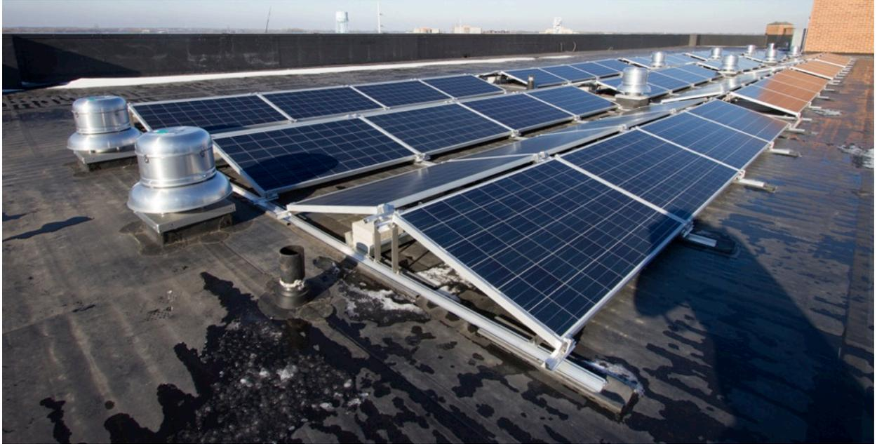
*Using SunPeak's exclusive east-west mounting system, self-shading was eliminated. This resulted in enhanced energy production per unit area on the small rooftop. Additionally, due to the aerodynamic nature of the design, wind resilience and long-term reliability were improved.*
